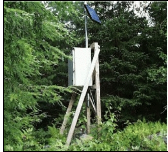
Solar-powered “Hydolab” water monitoring station on the Shelburne River.
