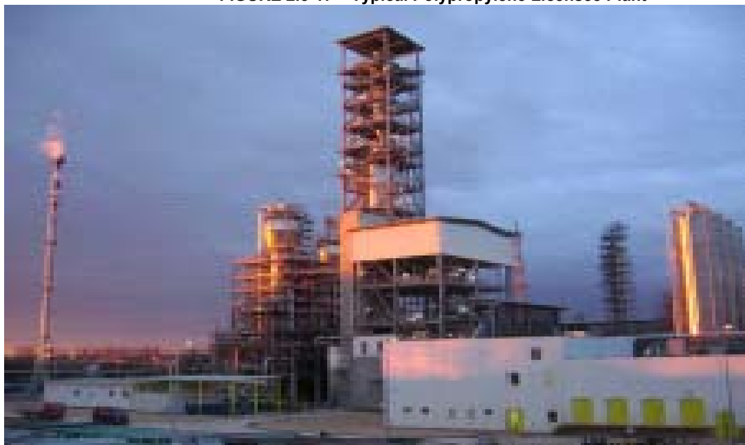
FIGURE 2.5-17 Typical Polypropylene Licensee Plant
