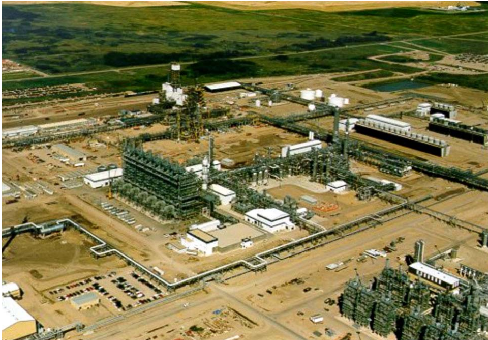
FIGURE 2.5-11 Typical Cracking Furnaces
