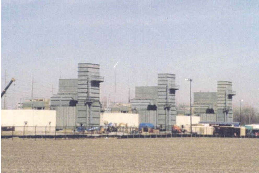
FIGURE 2.5-21 Typical View of Gas Fired Simple Cycle General Electric Frame 7EA Combustion Turbine Generators
