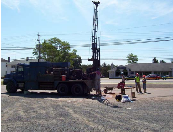
Photo 5: Drilling of MW 3 at south end of property.
