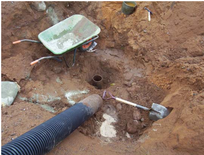
Photo 8: Drilled well casing exposed during excavation operations.
