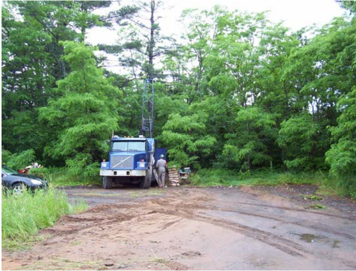
Photo 7: Drilling of MW 1 at north end of property.
