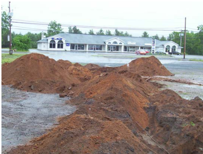
Photo 10: Extent of excavation area along eastern portion of property.
