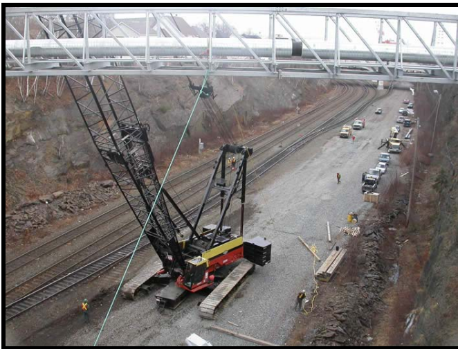
Halifax Harbour Solutions—Work in Progress
