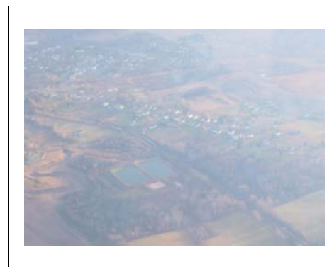
Hantsport Wastewater Treatment Facility
