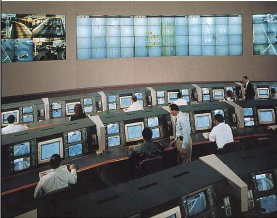
The primary objective of a CCTV camera is to provide surveillance of freeway / highway segments or intersections and visual confirmation of incidents, however it may also be used to detect incidents. A secondary benefit is the monitoring of environmental conditions including precipitation and visibility. CCTV supports other applications including vehicle classification and enforcement.
