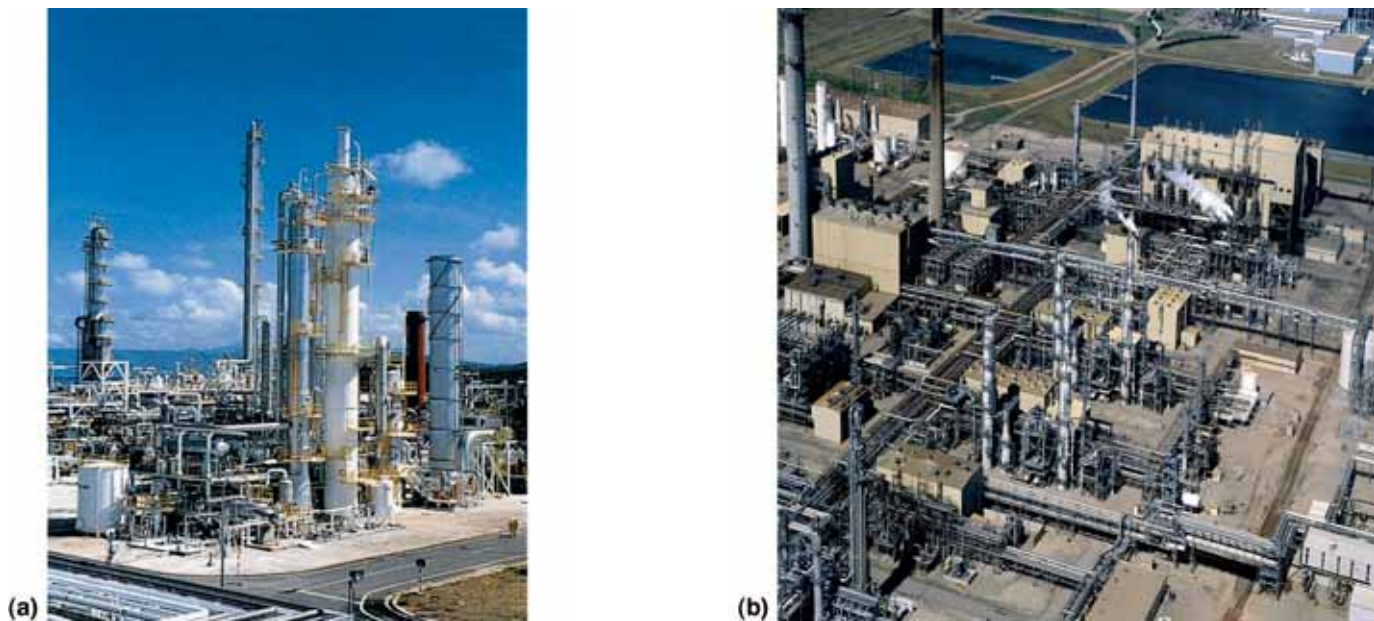
Figure TS.4. (a) CO 2 post-combustion capture at a plant in Malaysia. This plant employs a chemical absorption process to separate 0.2 MtCO 2 per year from the flue gas stream of a gas-fired power plant for urea production (Courtesy of Mitsubishi Heavy Industries). (b) CO 2 pre-combustion capture at a coal gasification plant in North Dakota, USA. This plant employs a physical solvent process to separate 3.3 MtCO 2 per year from a gas stream to produce synthetic natural gas. Part of the captured CO 2 is used for an EOR project in Canada.
