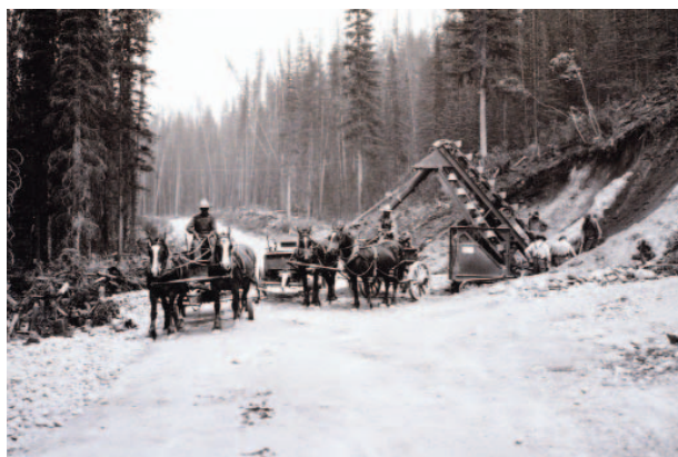
Road construction at Marble Canyon, Banff-Windermere Highway Kootenay NP of Canada (B.C.) © Parks Canada PHOTO: Parks Canada
