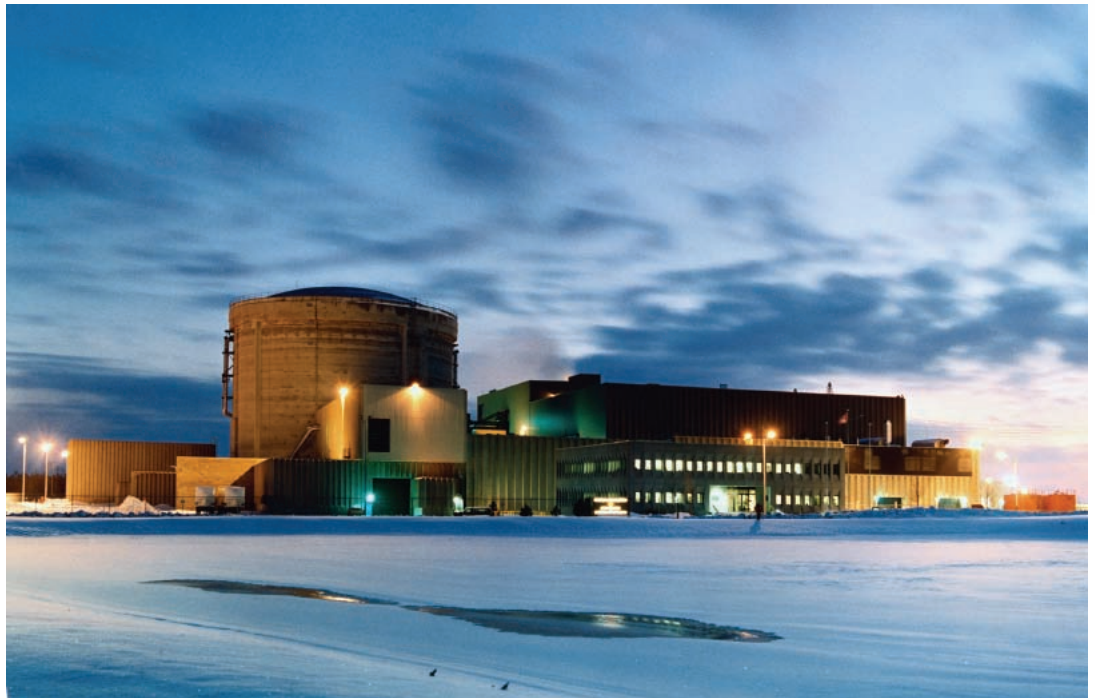
Point Lepreau Nuclear Generating Station, New Brunswick, Canada - in service since 1983
