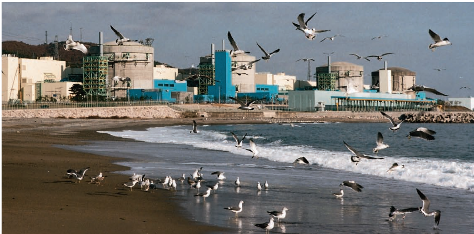
The Wolsong site in Korea: Unit 1 began operating in 1983 and is still a top-performing reactor. Unit 2 began operating in 1997, Unit 3 in 1998, and Unit 4 in 1999.
