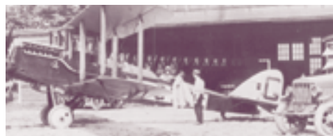
An Air Board de Havilland DH-4 aircraft preparing for an airmail flight to Toronto in 1923. By 1922 the canvas covering of the original hangar had been replaced with wood because of deterioration caused by the Canadian climate. (Public Archives of Canada PA 62293)
