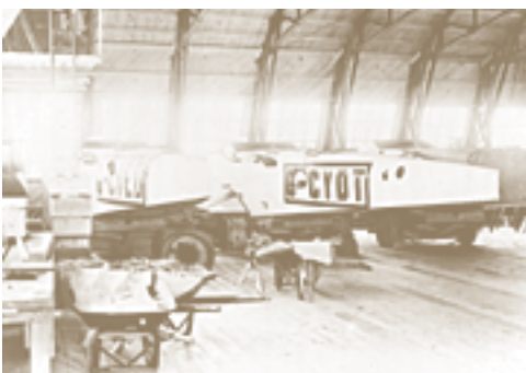
Interior view of the wooden hangar and hull of Curtiss HS-2L flying boat, Rockcliffe, 1922. (Public Archives of Canada PA 62292)
