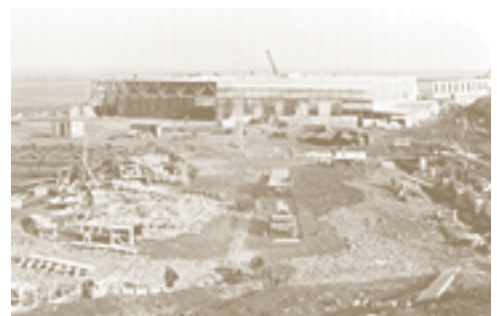
Construction of three more hangars on the south side of the field in 1942. The National Aeronautical Collection moved into these buildings after 1964. (Public Archives of Canada PA 64124)
