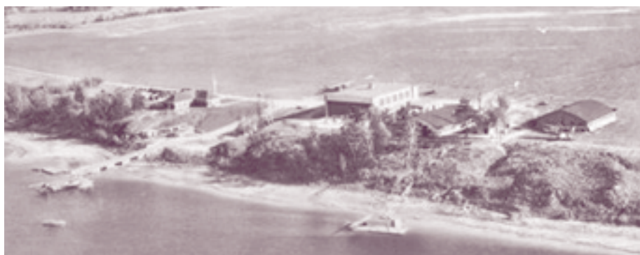
In this aerial photo of Rockcliffe taken around 1930, the new slipway and hangar built in 1928 are prominent while the old hangar is dwarfed beside it. (Department of National Defence RE 68-907)
