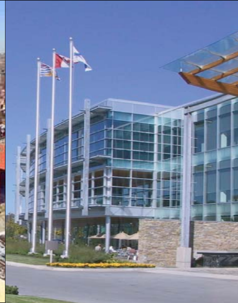
GLENLYON BUSINESS PARK VANCOUVER
