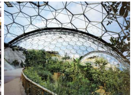
Eden House Project Greenhouse, Cornwall, UK Serre du projet Eden House, Cornwall, Grande-Bretagne 4
