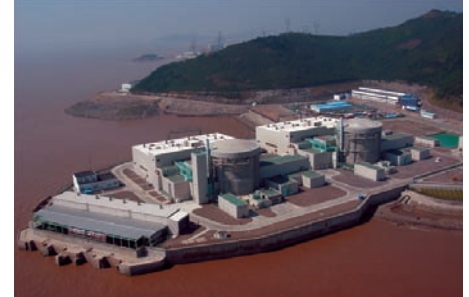
Qinshan Phase III, China, Units 1 & 2
