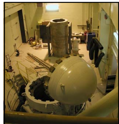
The Molten Fuel Moderator Injection Program investigates the potential impact of a severe accident scenario.
