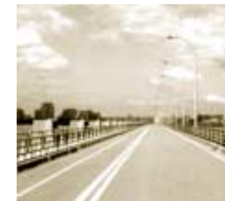
The Champlain Bridge Ice Control Structure
