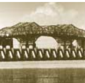
The Champlain Bridge and the Bonaventure Expressway
