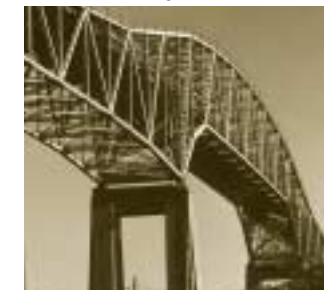
The Seaway International Bridge
