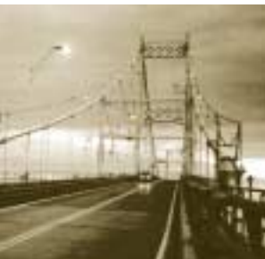
The Thousand Islands International Bridge
