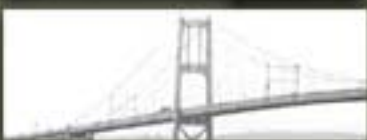
THE THOUSAND ISLANDS INTERNATIONAL BRIDGE
