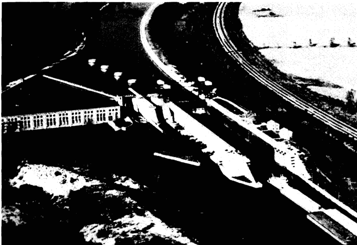
The Lake Michigan Diversion at Chicago is part of one of the most heavily used navigation systems in the United States.
