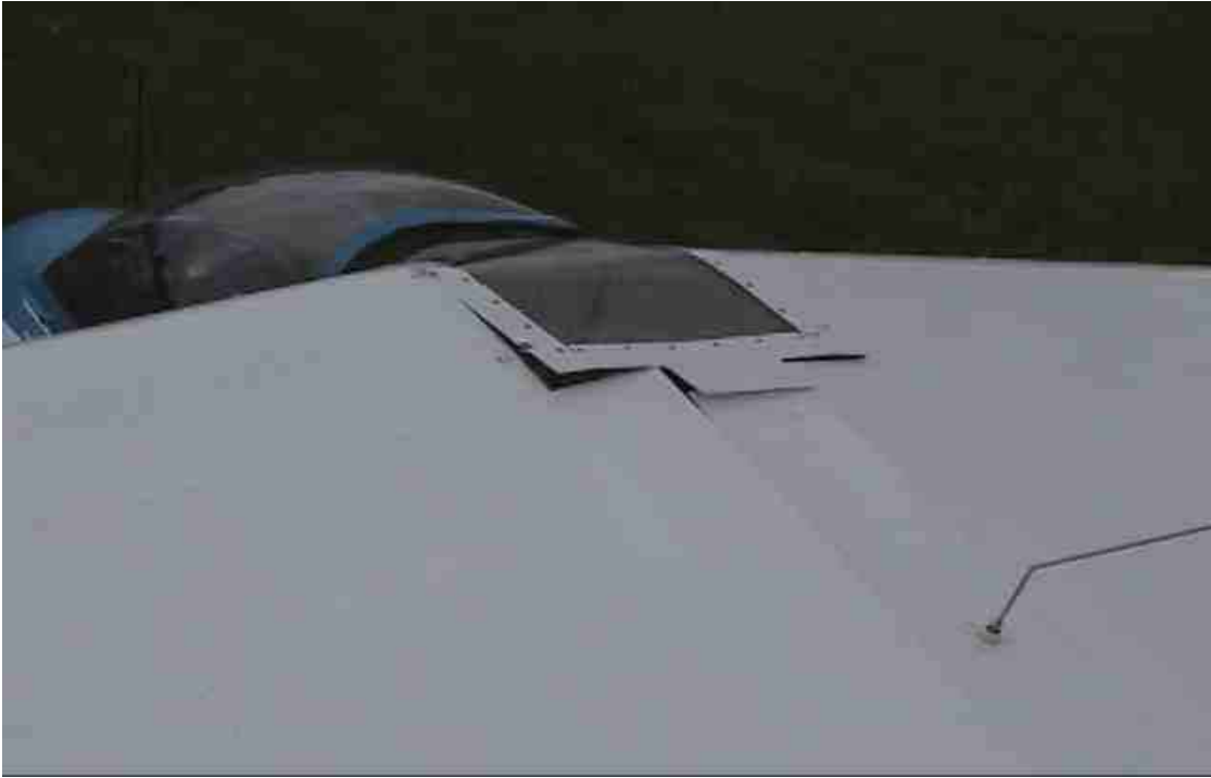
Top view showing skin buckling
