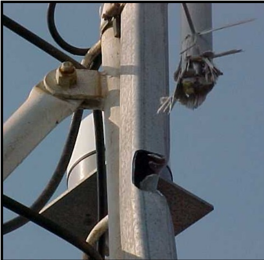
Photo 2: Stanchion and Antenna Damage
