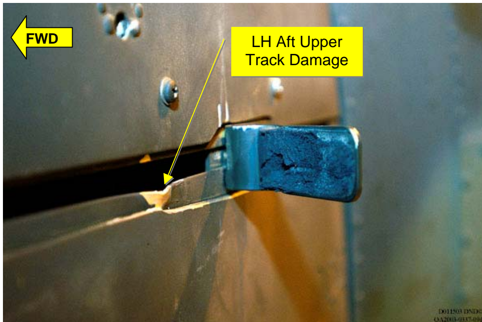
PHOTO 8 LH aft upper track damage consistent with the upper support roller being pulled from the track during the departure of the cargo door.
