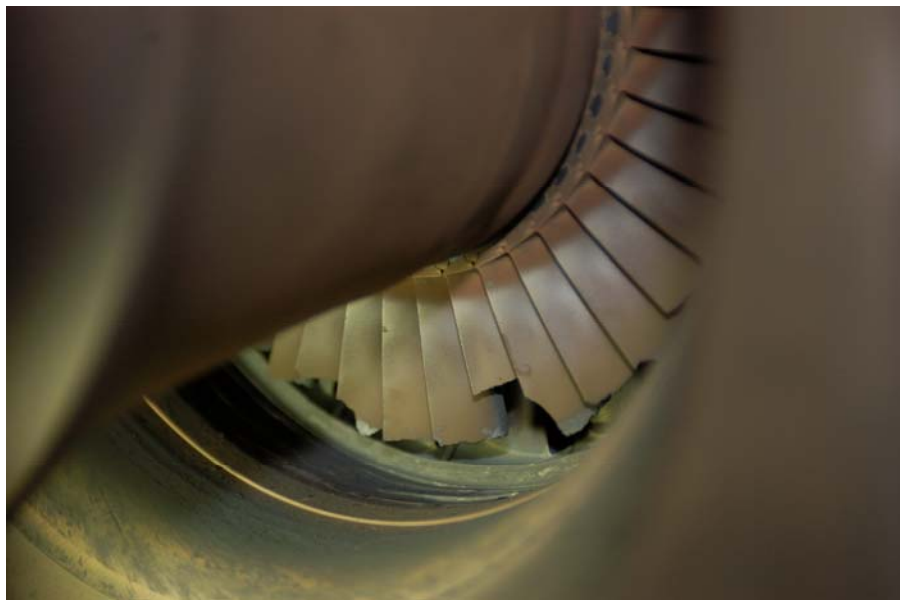
Photo 2: Number two engine, showing blade damage to the second stage of Power Turbine, as seen through the exhaust.
