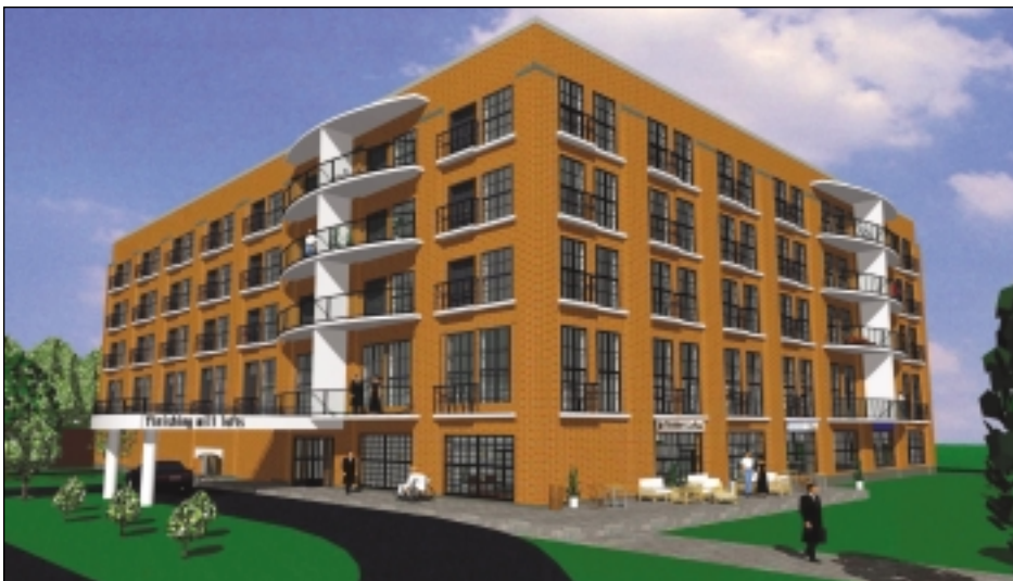
New finishing mill residential lofts
