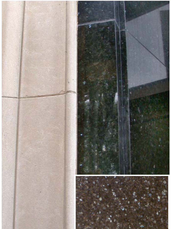
A view of the south entrance to the building reveals the use of Indiana limestone and black granite (close-up of the black granite with the blue crystals).
