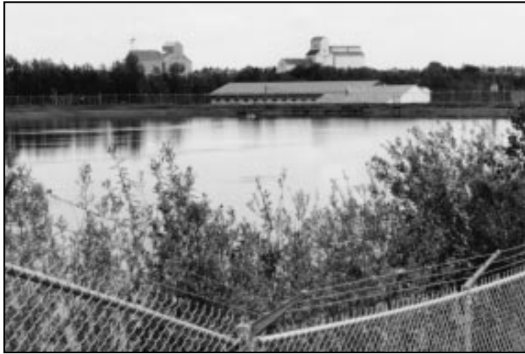
RAW WATER RESERVOIR
