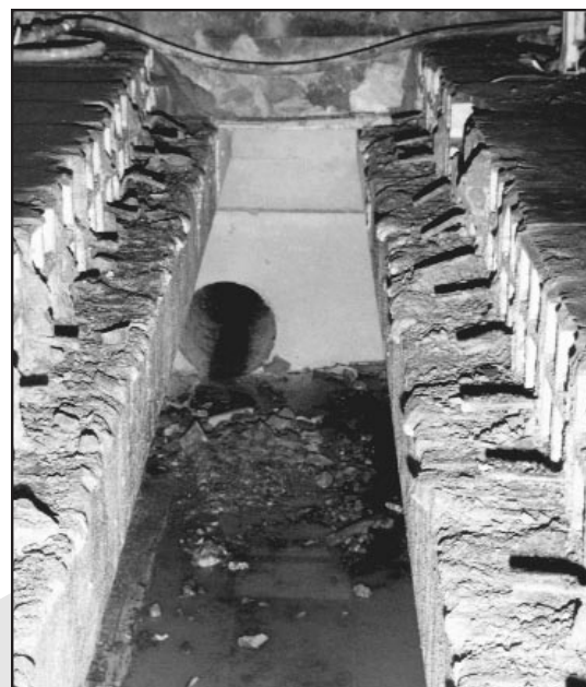
LEOPOLD BLOCKS AND EFFLUENT PIPE FROM FILTERS DURING FILTER REFIT
