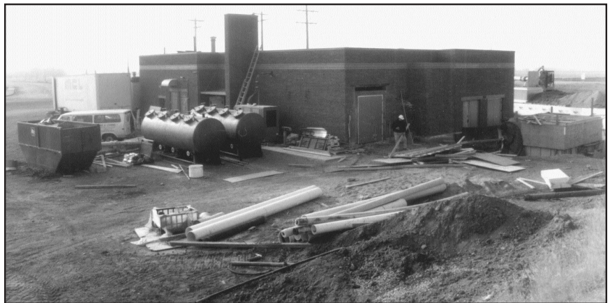
WATER TREATMENT PLANT UPGRADE OCTOBER 2001
