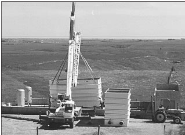
DAF PLANT UNDER CONSTRUCTION
