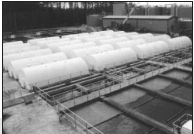
GRANDE PRAIRIE WASTEWATER TREATMENT FACILITIES
