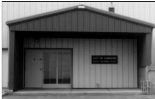
City of Camrose Water Treatment Plant
