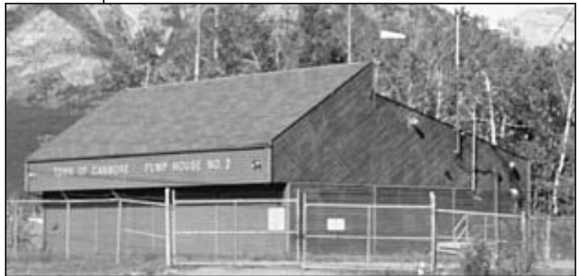
CANMORE PUMP HOUSE NO. 2 WATER TREATMENT FACILITY
