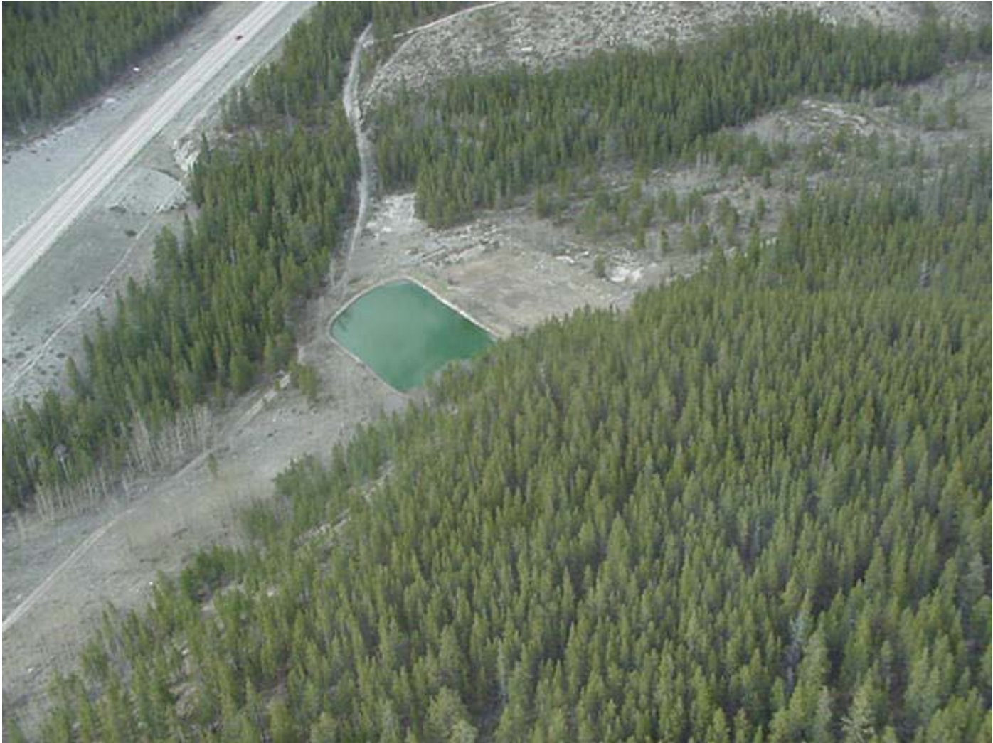
Existing Sewage Lagoon - David Thompson Resort
