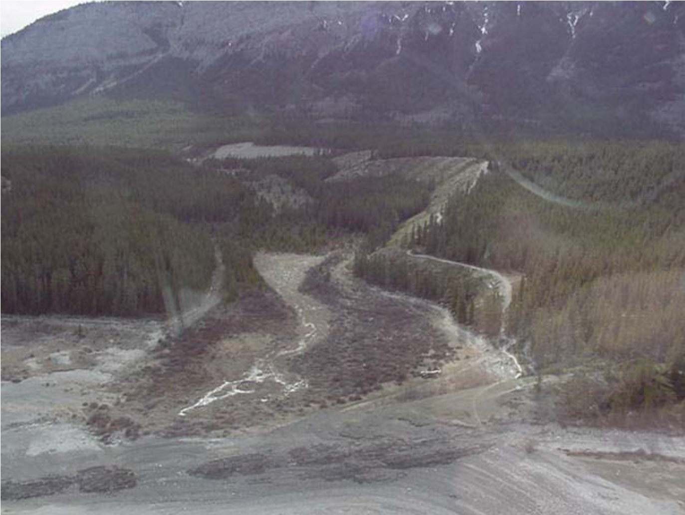
Creek between Development Areas - Sewage Lagoon Discharge Point
