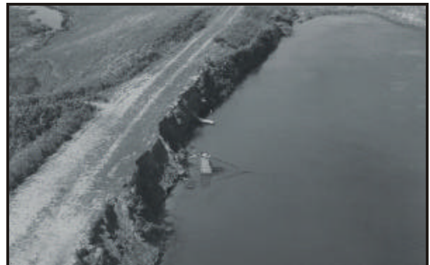
Photo No. 7 (DSB 7823-24A) Extensive erosion of the upstream slope caused by wave action. This has displaced all the riprap, created beaching and vertical scarps, reduced crest width and left the riparian outlet control unsupported.
