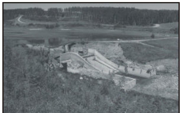
An overtopping failure as a result of storm runoff larger the spillway capacity.
