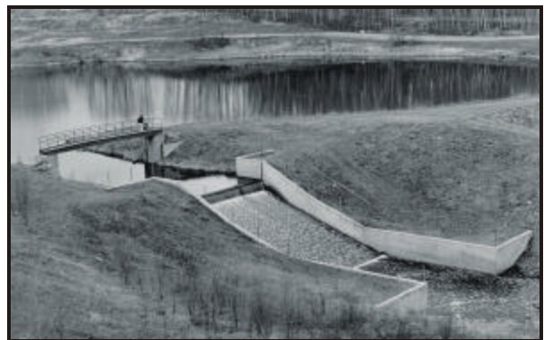
Photo No. 1 (DSB 8609-19) Mound Red Park Reservoir – 1986
