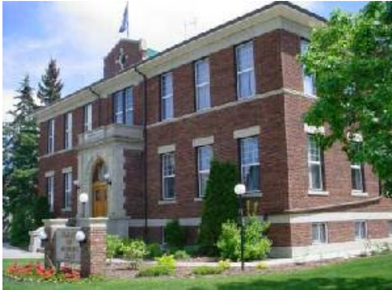
The County of Minburn No. 27 moved into its Administrative Complex in 1991. This building--acquired from the provincial government [old courthouse] and renovated--preserves the historic link to the past.
