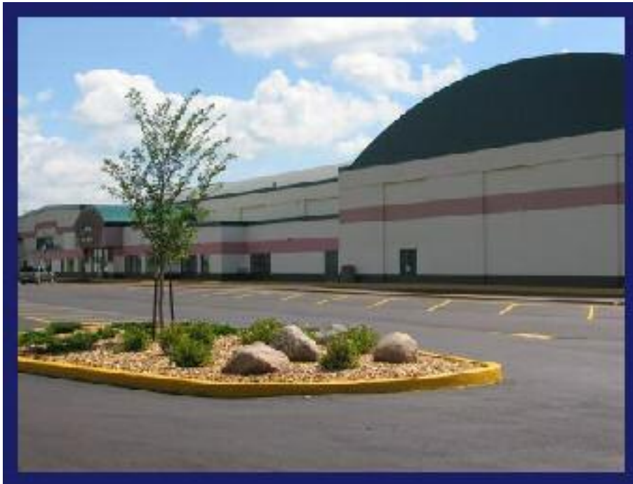
Wetaskiwin Civic Centre Drill Hall, Arena I & Arena II
