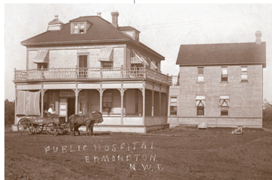
Provincial Archives of Alberta, A2994 Public Hospital – in operation between 1900 - 1911
