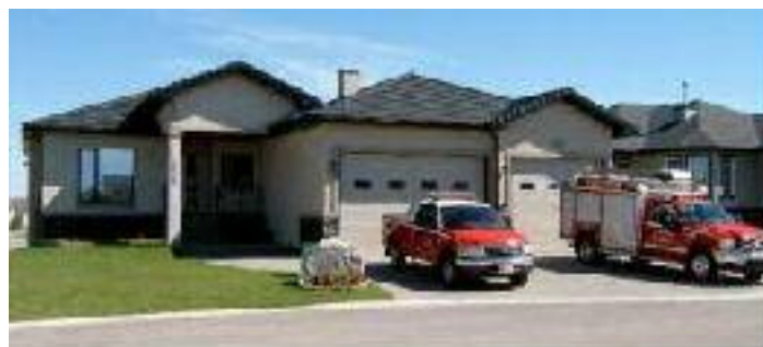
High River's Fire House
