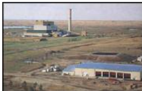
Luscar shop facilities with Sheerness Generating Station in the background.
