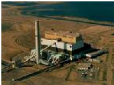
Sheerness Generating Station
