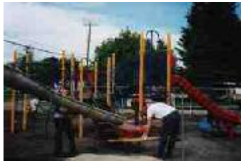
Alliance volunteers construct a new playground for the primary school.
