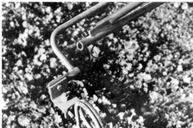
FIGURE 18. Failed Boom End.
