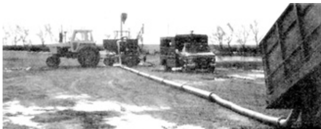
FIGURE 10. Inlet Length of 30.5 m.
