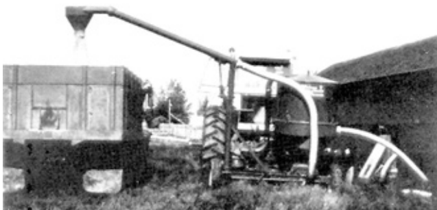
FIGURE 4. Bin Clean-out Nozzle Attachments.
