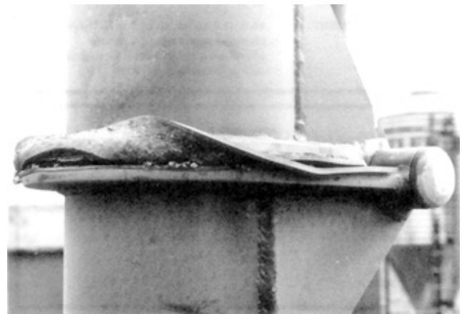
FIGURE 16. Seal Failure on Folding Discharge Boom.
