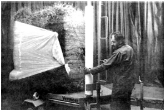
FIGURE 4. Applying Tension to Plastic Roll.
