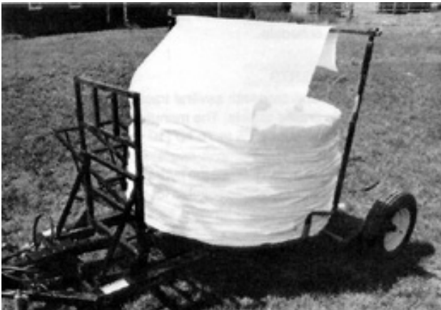
FIGURE 3. Installing Poly Tubing from Roll onto Drum.
