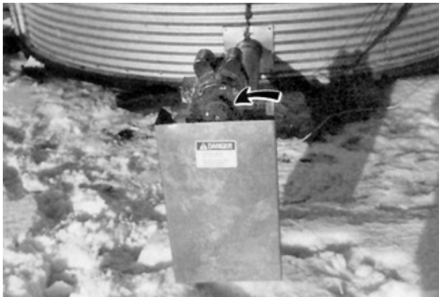
FIGURE 11. Exposed Discharge Auger Drive.
