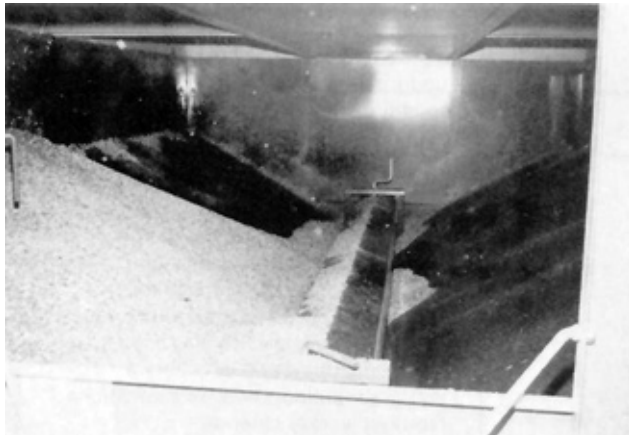
FIGURE 10. Buildup of Grain in the Dry Grain Holding Chamber.
