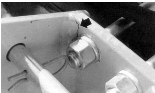
FIGURE 8. Shank Assembly Weld Cracks.
