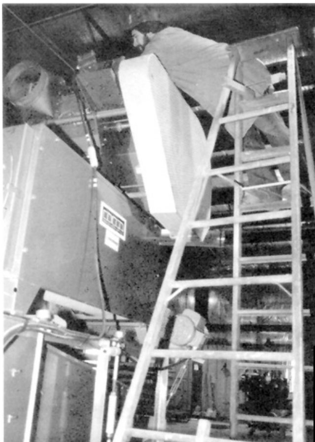
FIGURE 5. Adjusting Aspirator Controls.
