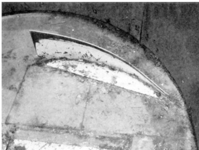
FIGURE 3. Fin on Tub Floor Repositioned.
