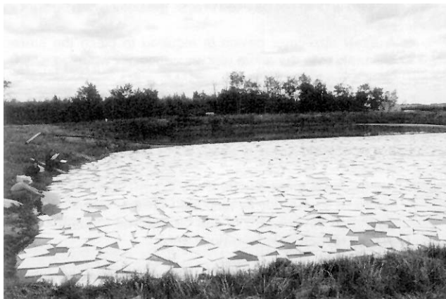
FIGURE 2. Floats in Place on Liquid Cell.
