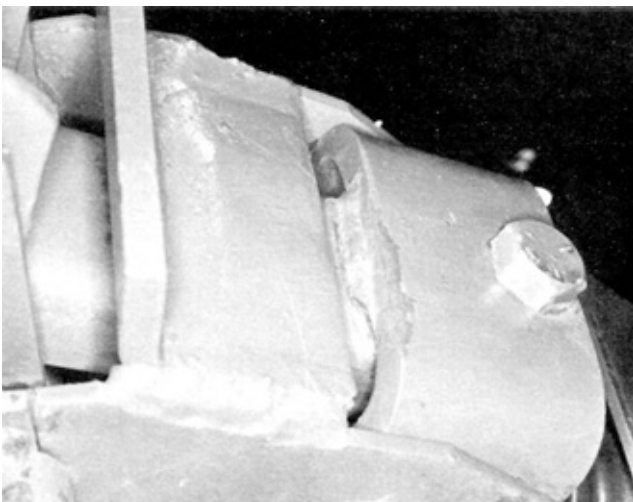
FIGURE 13. Shank Holder Cracks.
